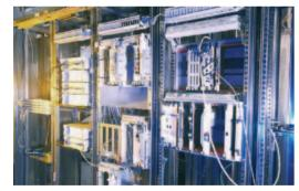
Fig. 3.1.4 Optical networks: Compact Add Drop Multiplexer and Mini Cross Connect for city networks/test and integration © Alcatel
