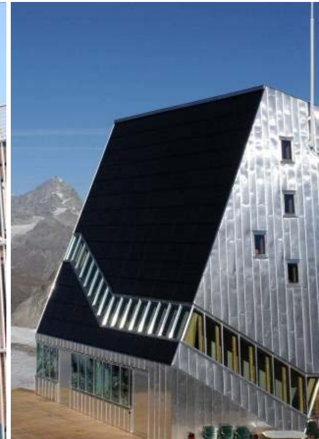
Solar façade „Monte Rosa“ High efficiency 3S glass/glass modules
