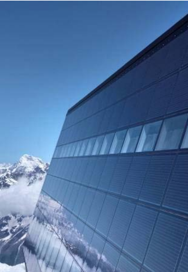
Solar façade „Kleines Matterhorn“ 3S glass/glass module applied in the Alps, 3'800m above sea level
