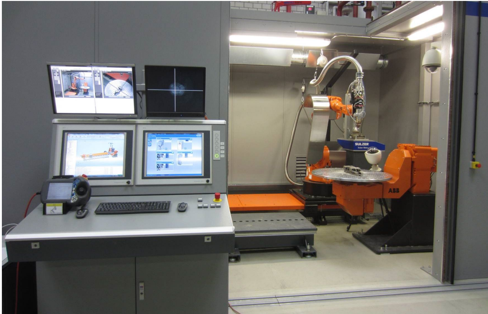
Operator desk with LC-Controller, offline programming system, camera surveillance and device monitoring tools
