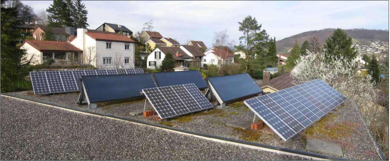
Figure 1: This solar installation in Frenkendorf BL is oriented exactly to the south even though the building points south-southeast.
