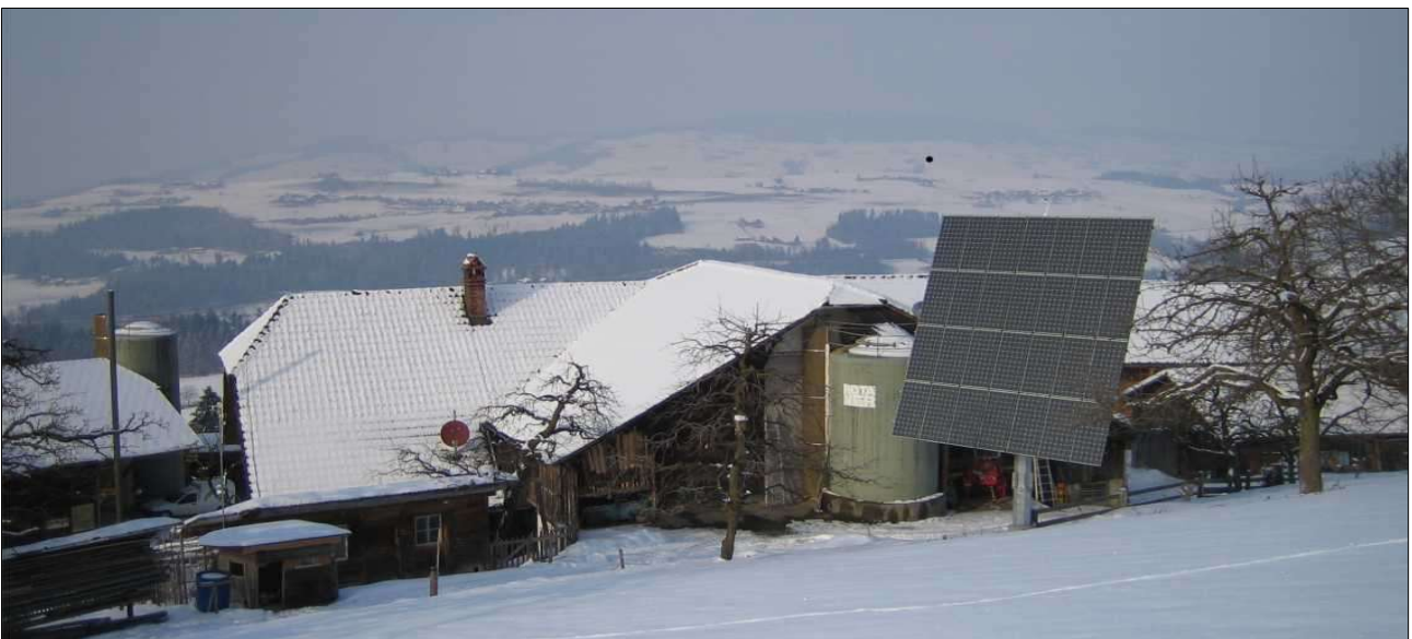
Figure 2: This installation in Schwendibach, Homberg, BE, always points directly to the sun.
