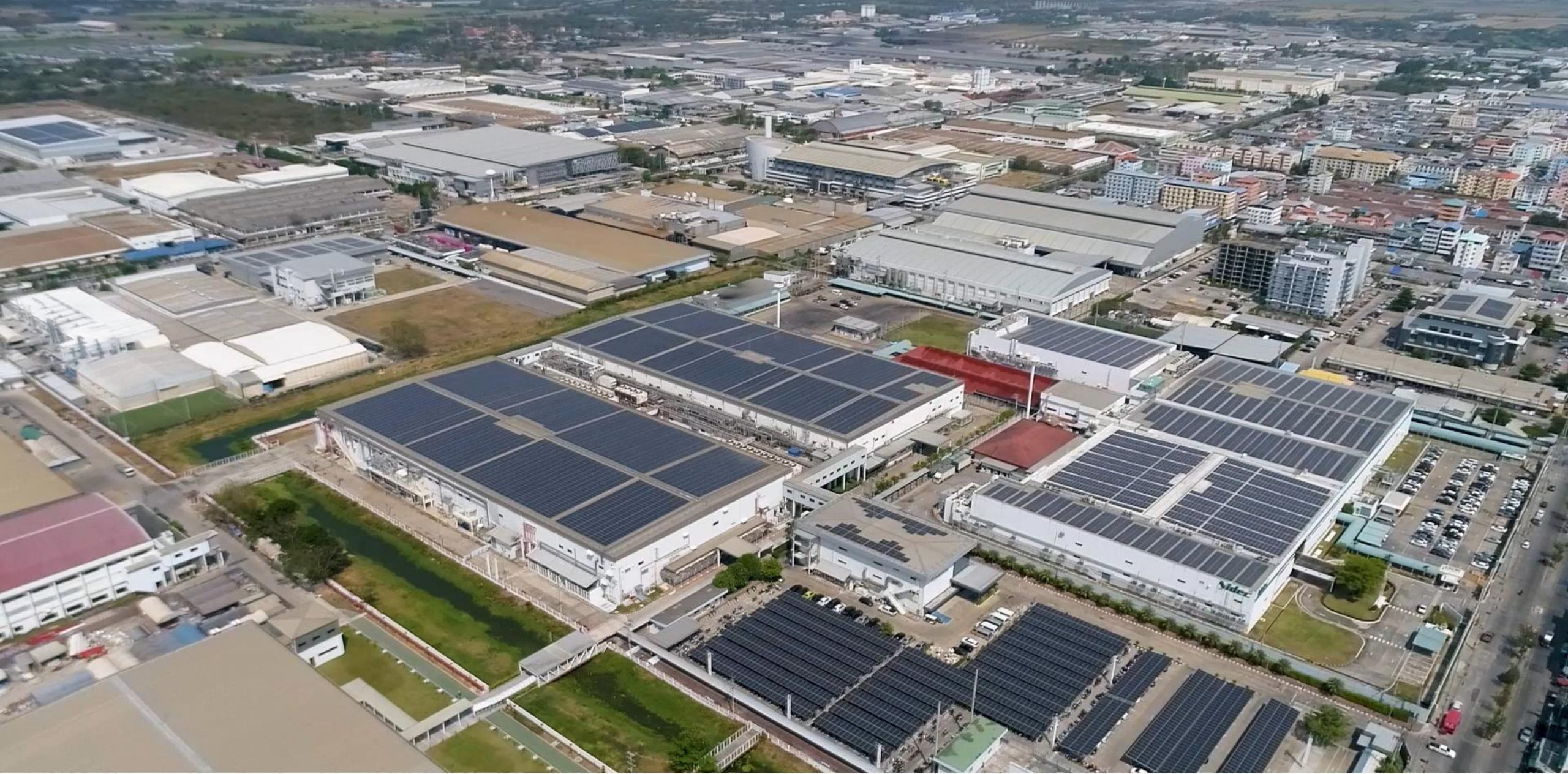
Navanakorn, Thailand 1.5M SF Manf. Facility
